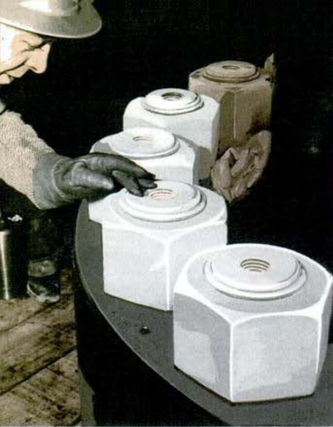
18 These huge nuts, used to couple the shaft of the waterwheel to the generator rotor, were shrunk with Dry Ice to 80 degrees below zero so they will expand and tighten after fitting
